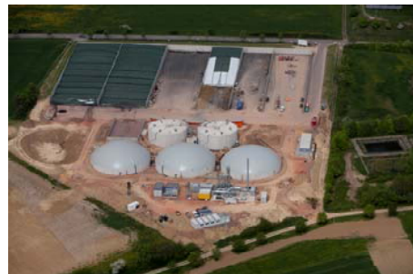
Merzig: 50 GWh/a in operation since 05/2011
