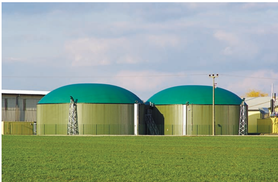
Figure 3-23: Typical farm-based vertical digester system
