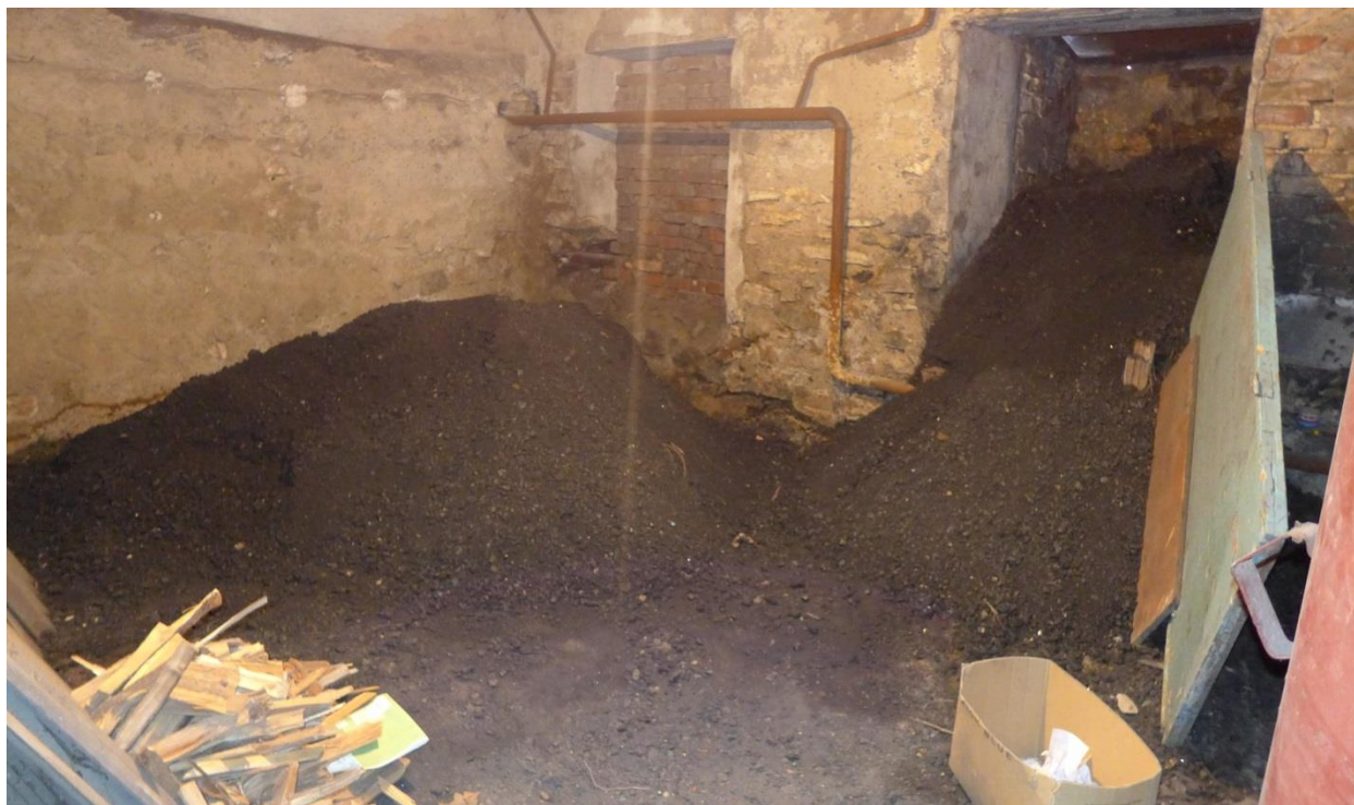
Coal storage bunker
