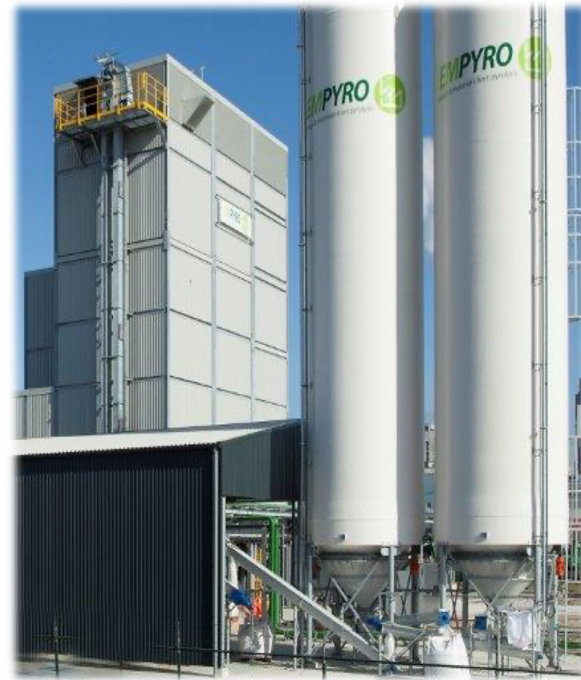
Empyro Hengelo Biorefinery (Netherlands)
