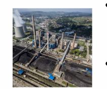
Co-firing of biomass (up to 30 % weight) with brown coal
