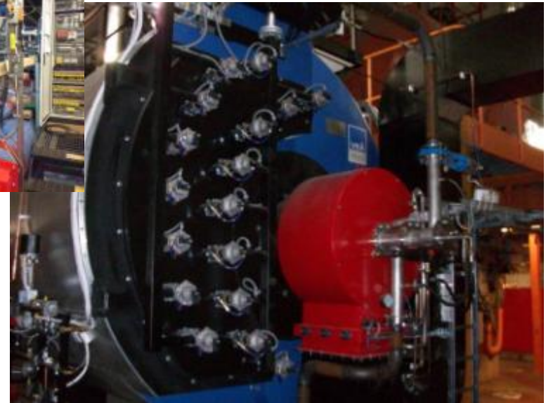
Horizontal furnace, fire-tube boilers
