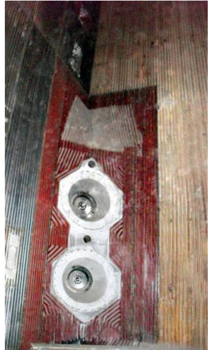
Burner configuration In the corners
