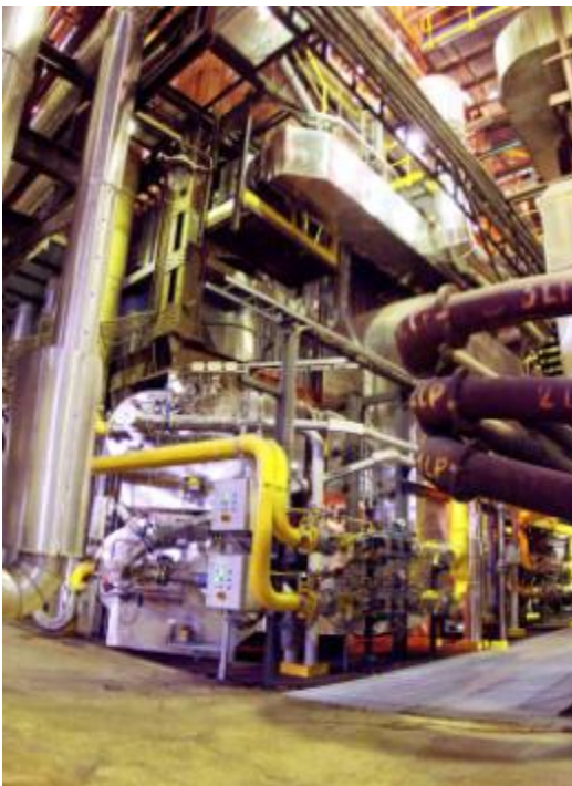
Water tube boiler CHP, tangential fired
