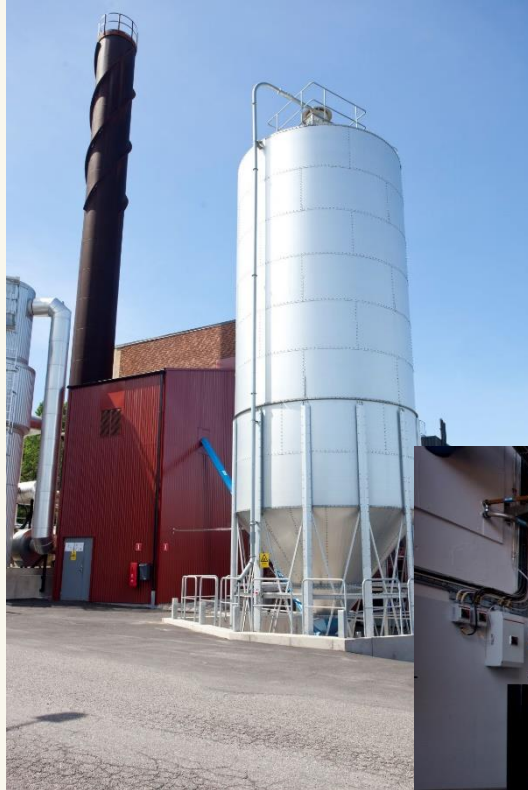
Fuel storage and milling house
