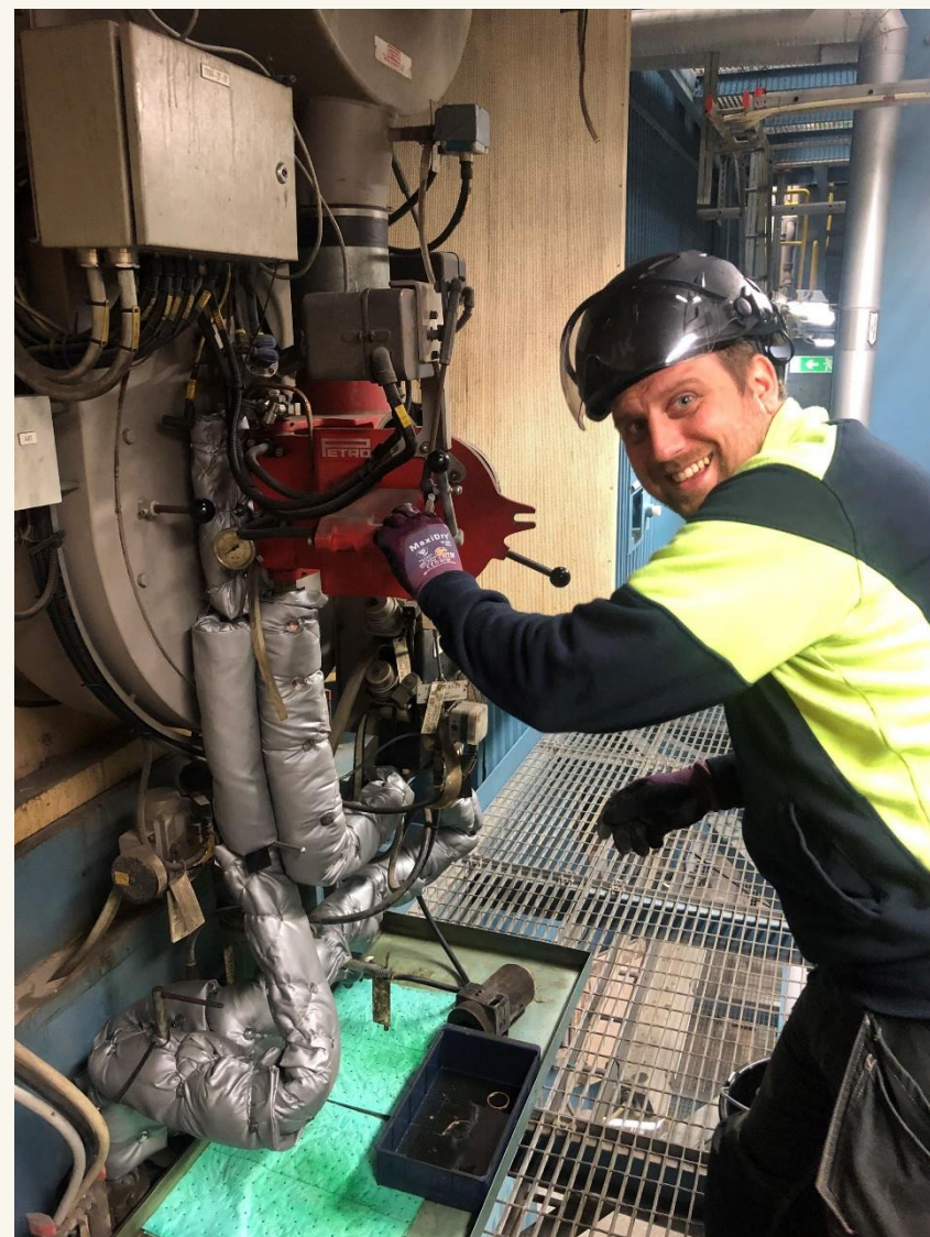
One of our commissioning engineers ready for start up of converted burners in a Waste to Energy boiler
