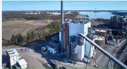
Multifuel to energy
