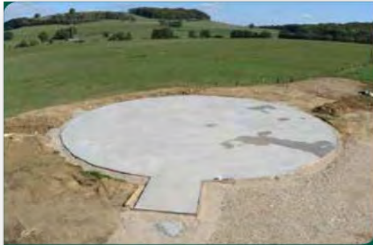
On-site base plate
