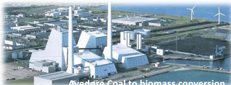
Avedøre Coal to biomass conversion
