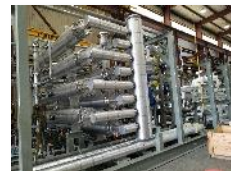
FABRICATION ASSEMBLY & TESTING
