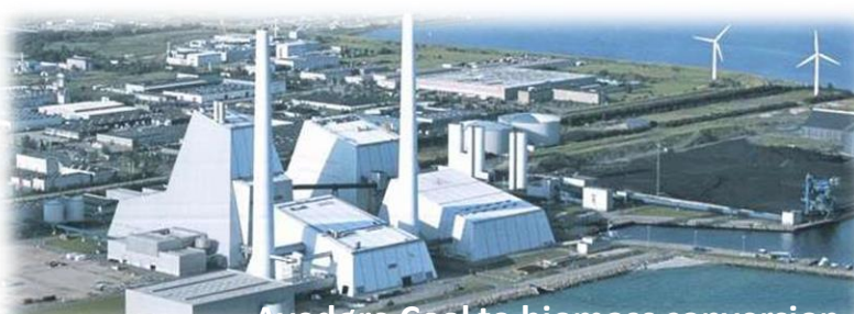
Avedøre Coal to biomass conversion
