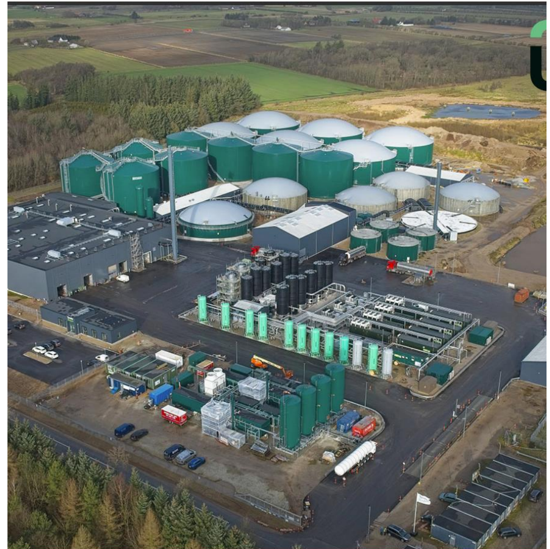
Tønder Biogas, January 2025
