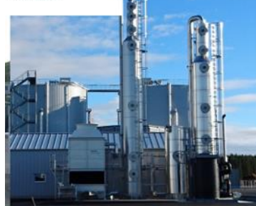
Biogas: 1300 Nm 3 /hr Bio-CH 4 : ~780 Nm 3 /hr ~ 77 GWh
