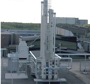
Biogas: 300 Nm 3 /hr Bio-CH 4 : ~180-Nm 3 /hr ~ 17 GWh
